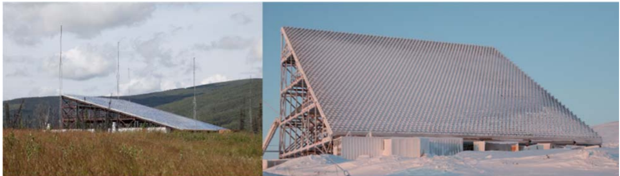
Figure 12. PFISR (left) and RISR-N (right) systems.
